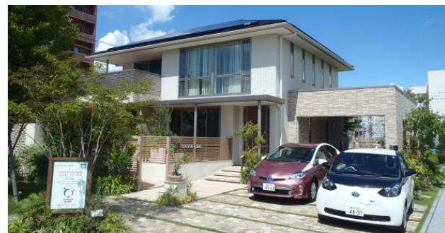
[A smart house connected with vehicles at Ecoful Town] A house with a solar power generation system, battery and HEMS and next-generation vehicles (left: PHV right: EV)
