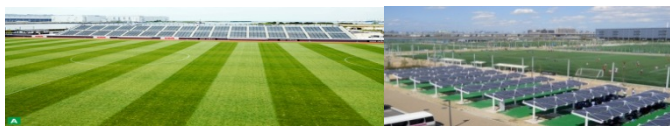
J-GREEN Sakai (Japan's biggest photovoltaic generation for a sports facility including soccer)
