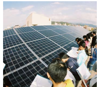
Viewing a photovoltaic system installed on the rooftop of an elementary school
